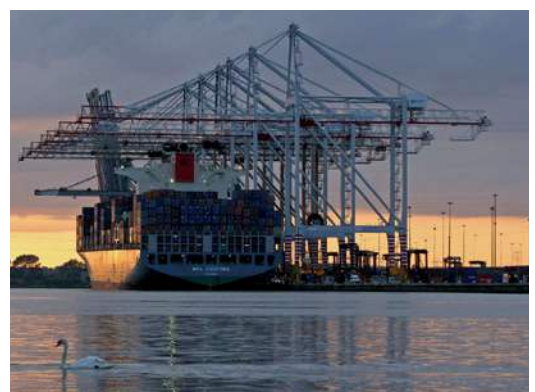
Ship to shore cranes.
