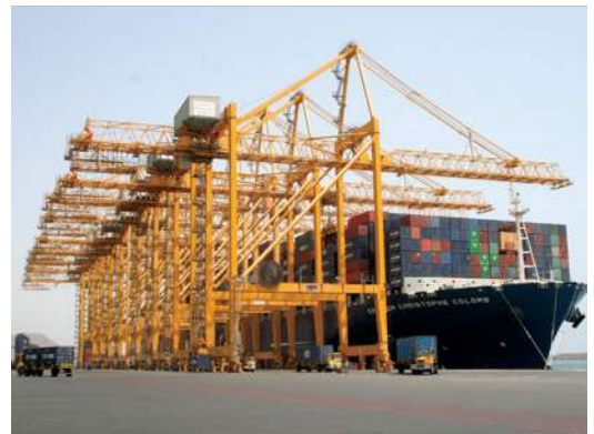
Ship to shore cranes.
